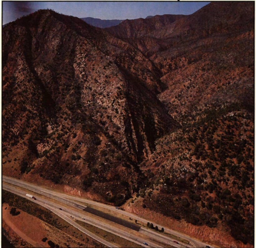
Photo 7. East drainage escape route.
